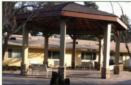
Generous donors to the Sunny View Foundation contributed to the construction of the new gazebo and brick walkway.
